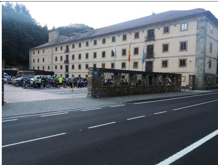
Our Hotel in Cangas – the Parador Nacional de Corias This is only one ¼ of the building – it's huge
